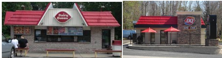
Before and after recent renovations
